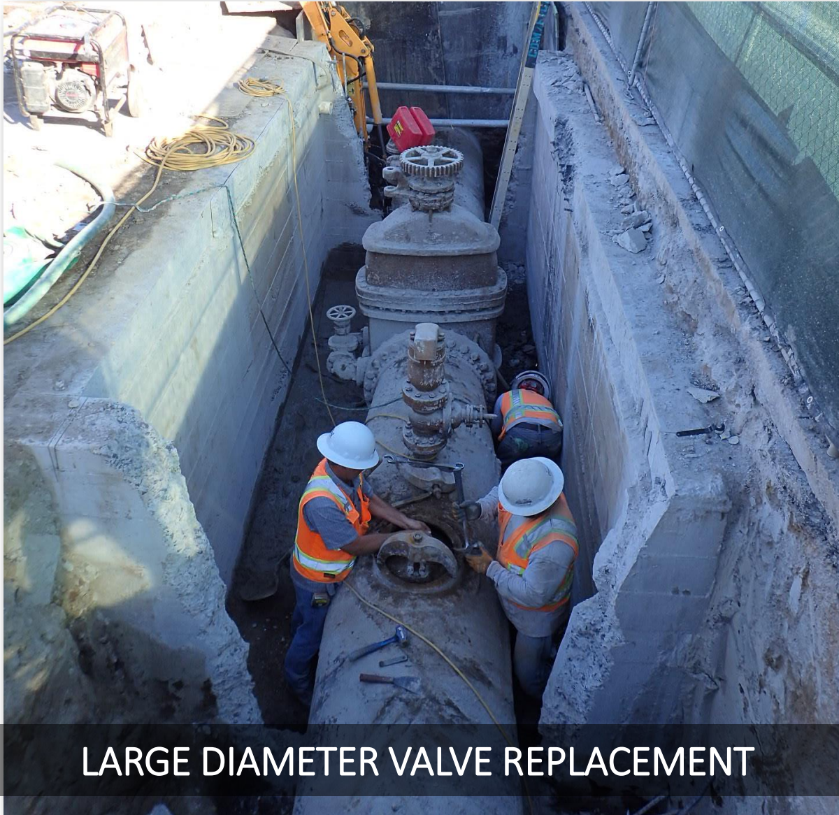
PIPELINE REPLACEMENT AT BRIDGE CROSSINGS
