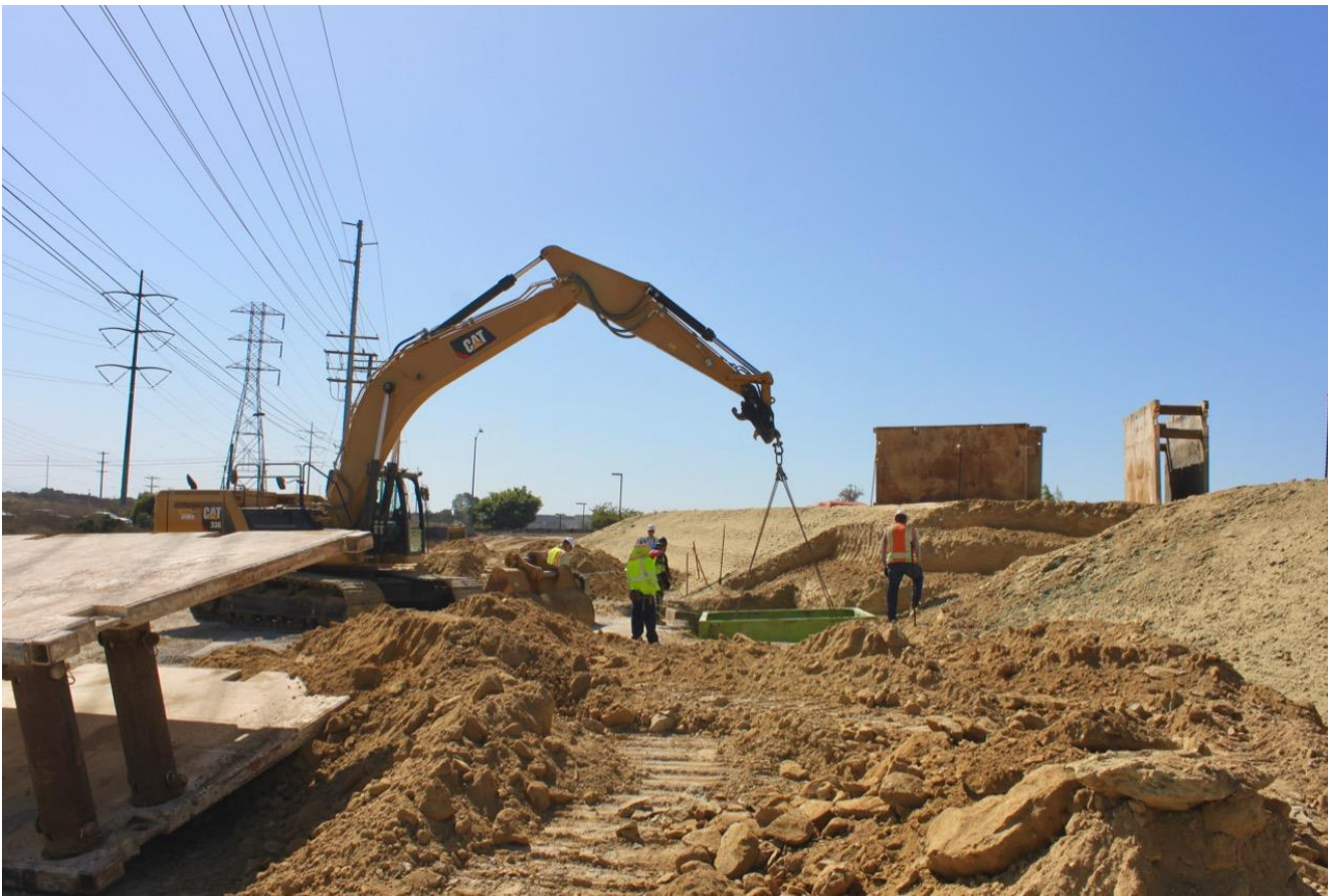
Early Site Work at the North City Water Reclamation Plant
