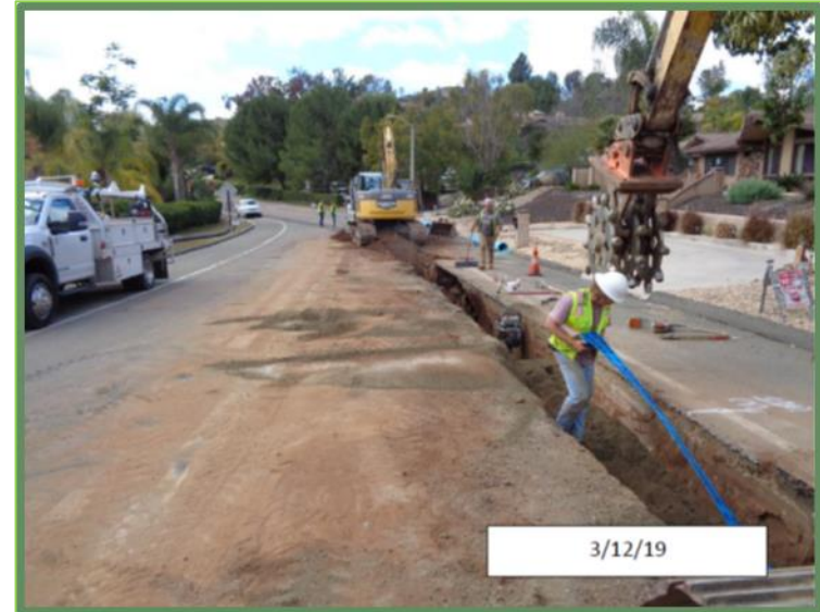
Water Main Replacement
