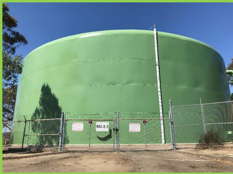
Reservoir Coating and Upgrades
