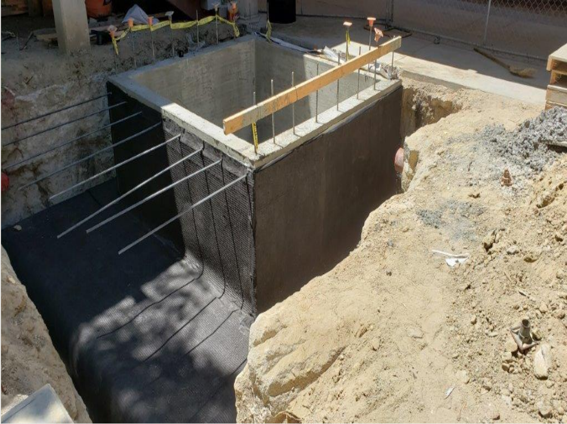
Frost Middle School New Elevators Project
