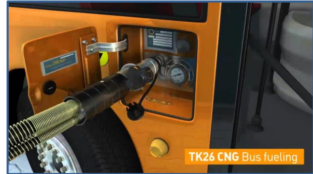
CNG Bus Fueling
