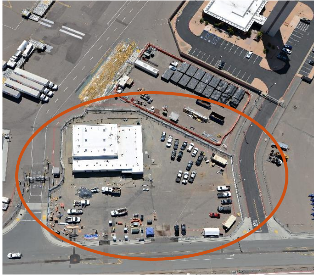
Aerial View of AFO site as of May 2020
