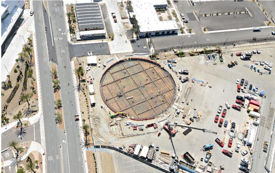
Construction progress as of May, 2020
