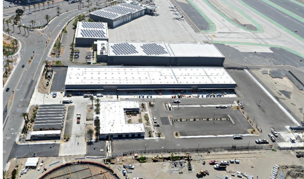
Construction Progress as of May 2020
