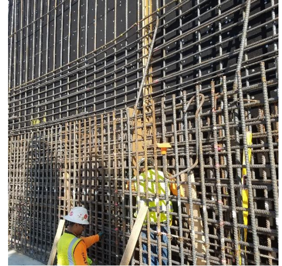
Tons (literally) of steel rebar being placed to allow concrete walls to withstand external pressure without cracking
