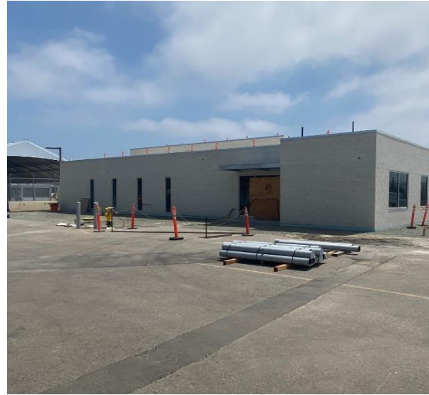
Finishing up Glazing and CMU Block Sealant on Administrative Portion of Building
