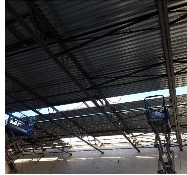
Installation of Roof Deck in Fuel Truck Maintenance Bays Area
