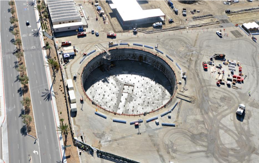
Construction progress as of January, 2020
