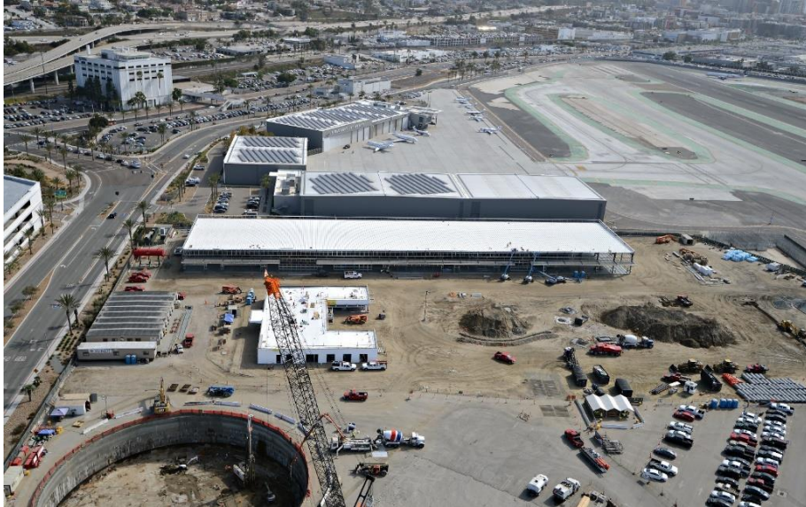
Construction Progress as of January 2020
