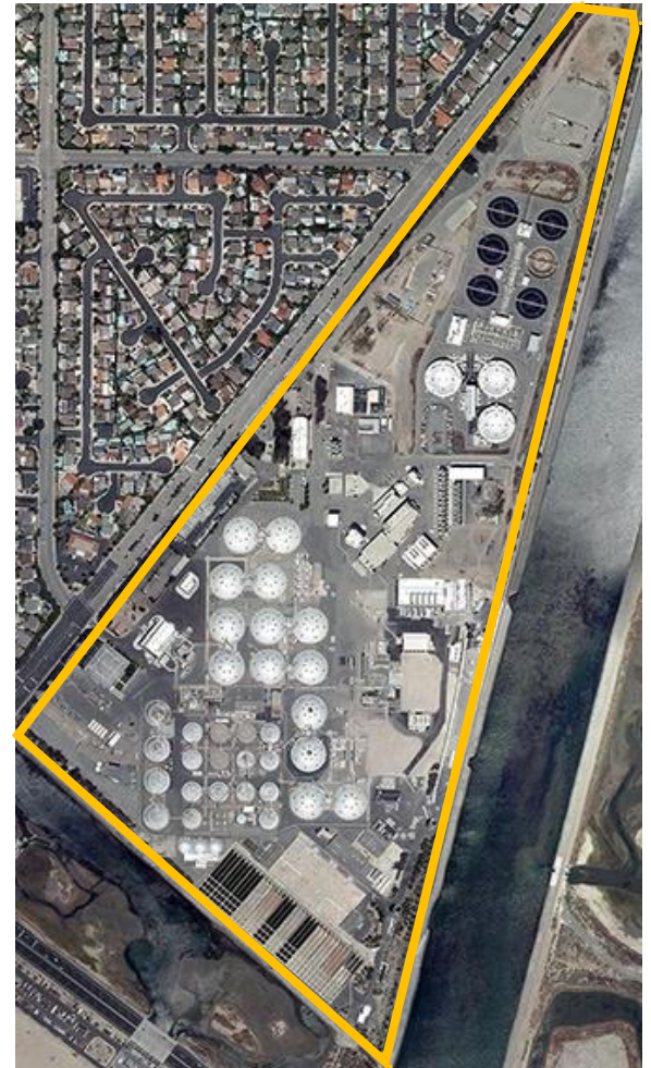
Treatment Plant No. 2 Huntington Beach
