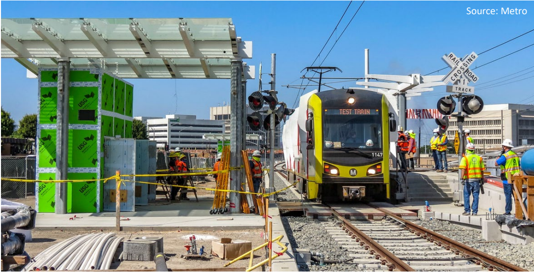
2014 – Construction Begins on the Metro Crenshaw/LAX Line
