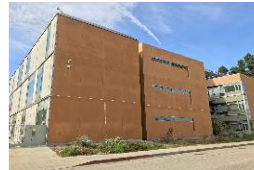
Allied Health and Science Center: Laboratory Wing Stucco Repair PQSP Project Completed in February 2021
