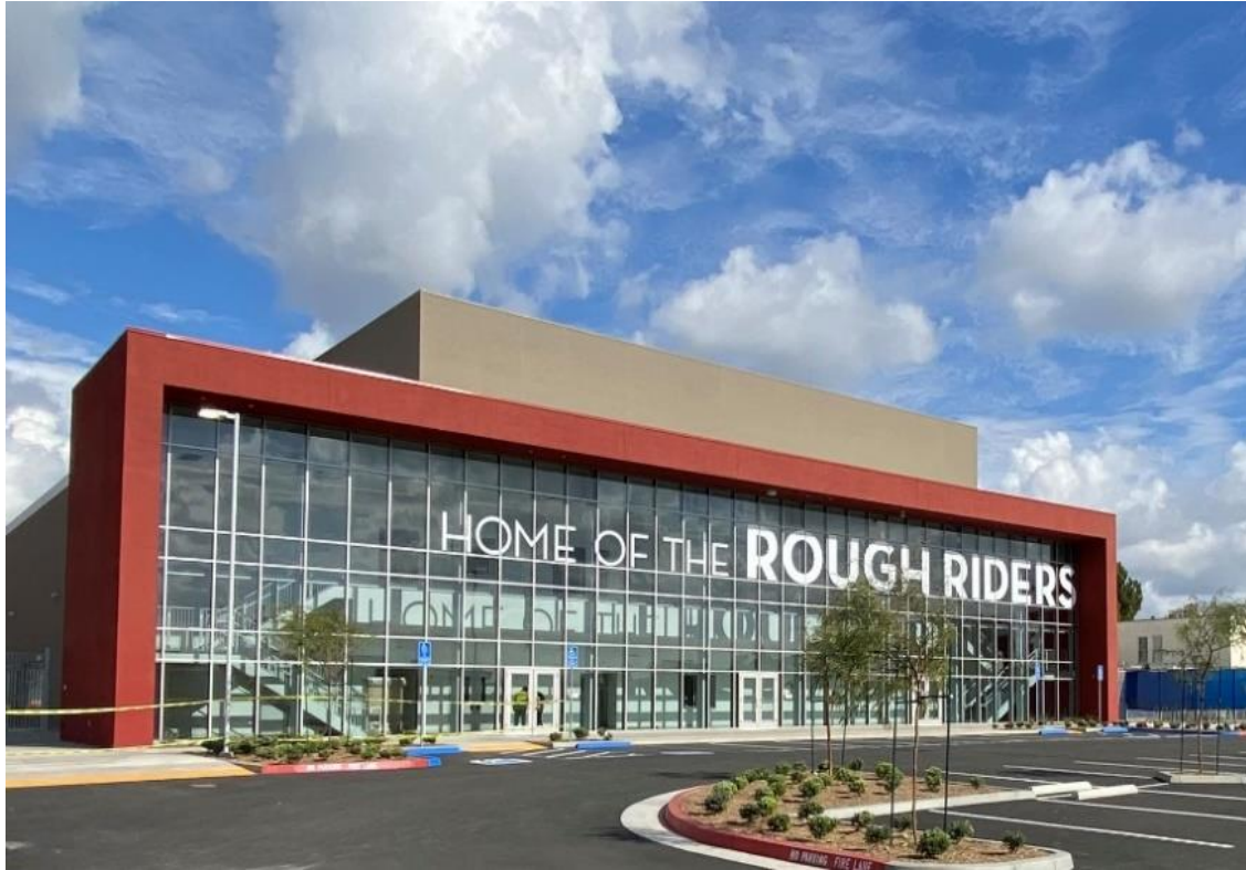
New Gymnasium Building
