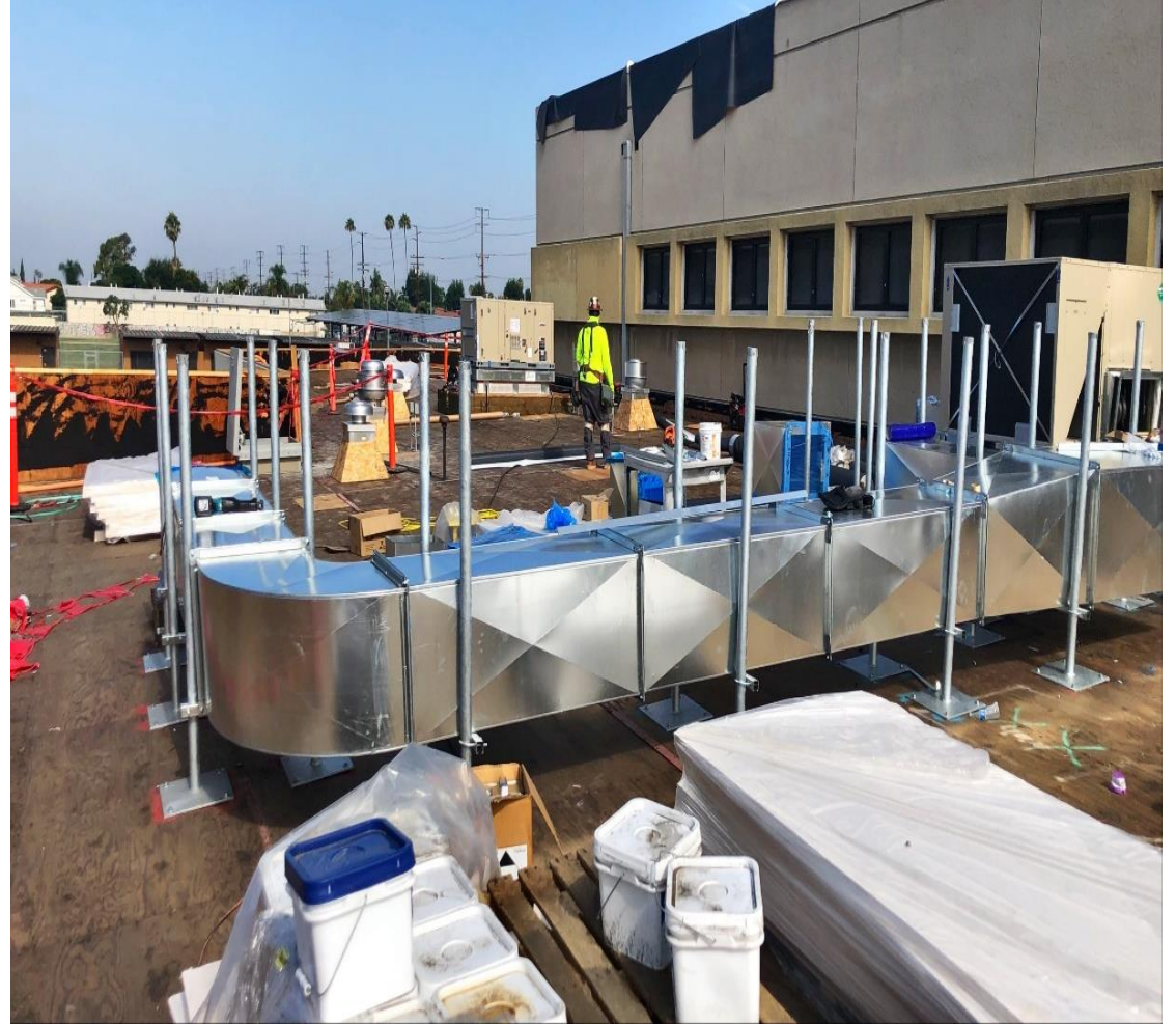
HVAC Duct and Unit Installation
