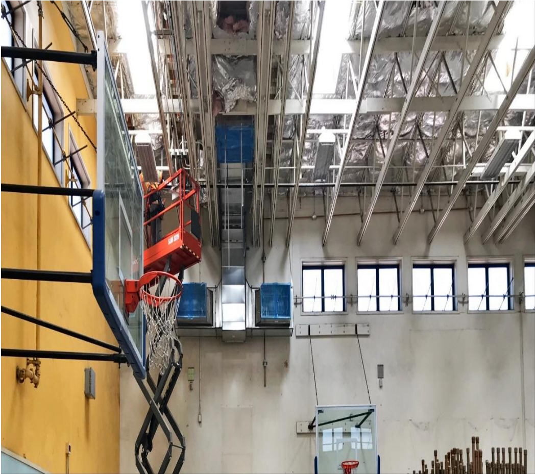
HVAC Duct Work in Gym
