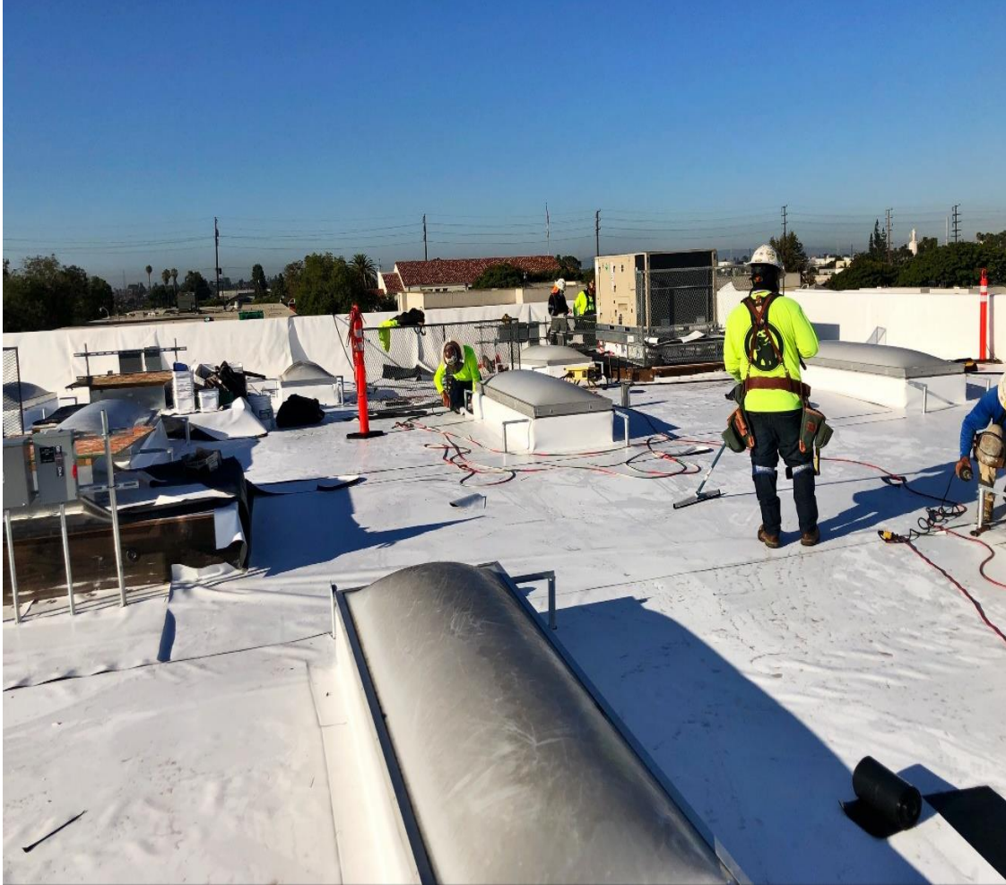
Gymnasium HVAC and Roof Installation
