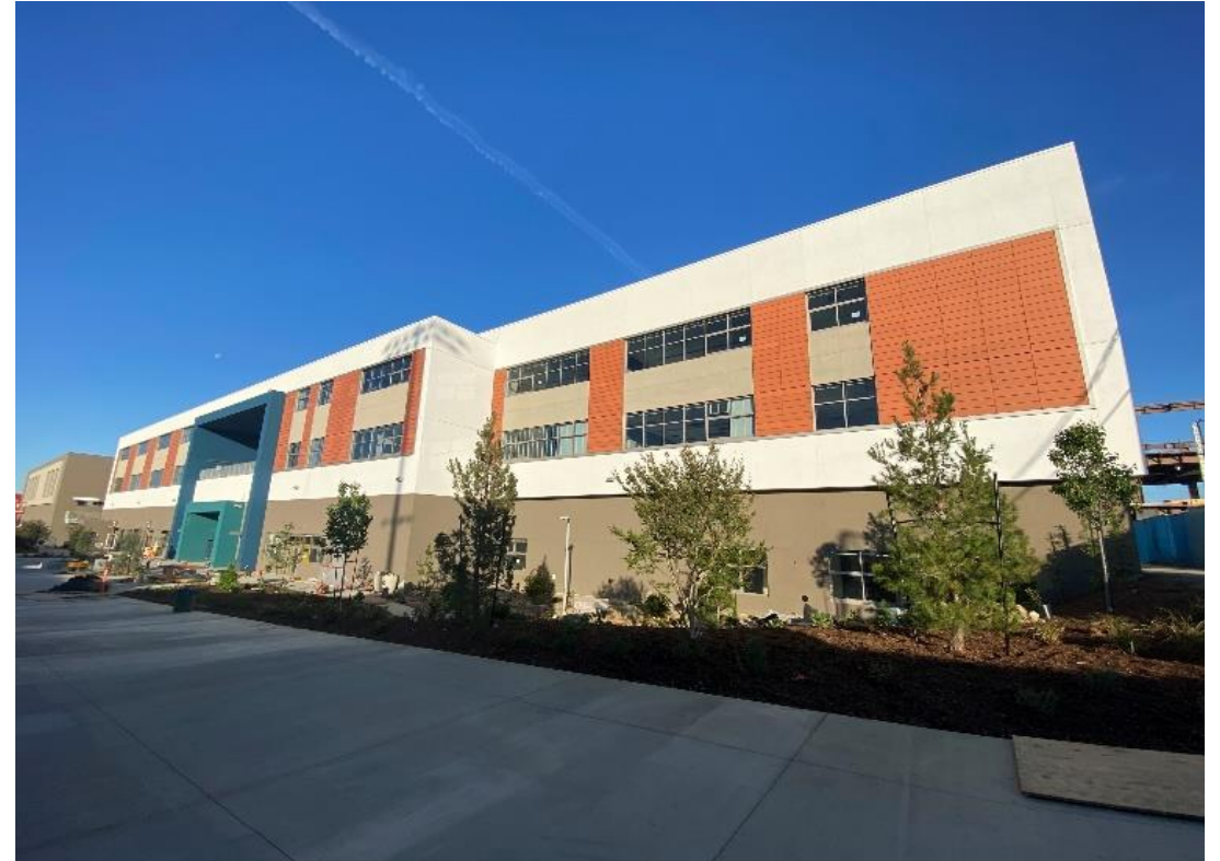
New Classroom Building
