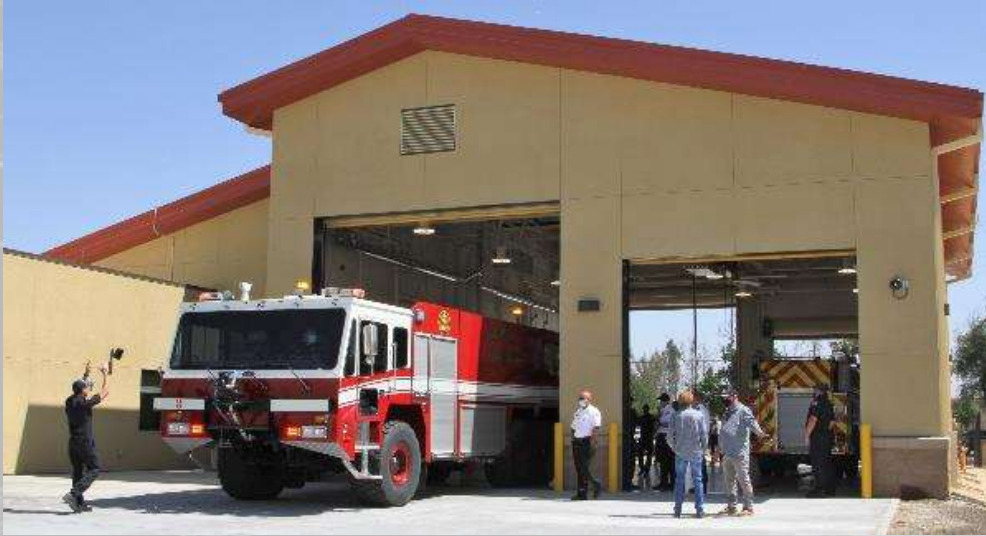
Newly constructed fire station at March AFB Spring 2021
