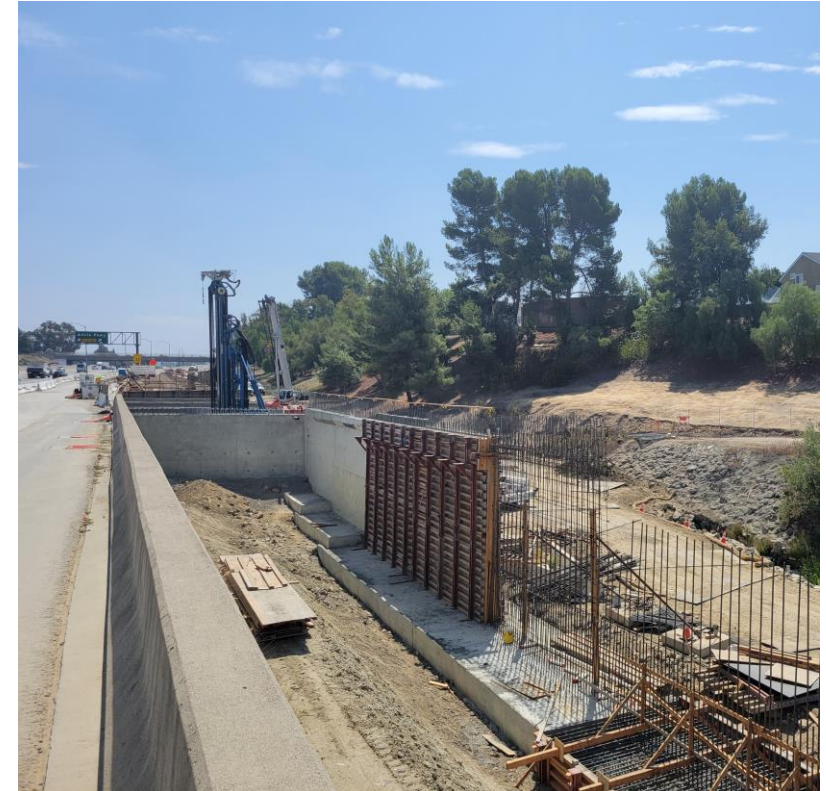
Aliso Creek bridge widening Segment 3
