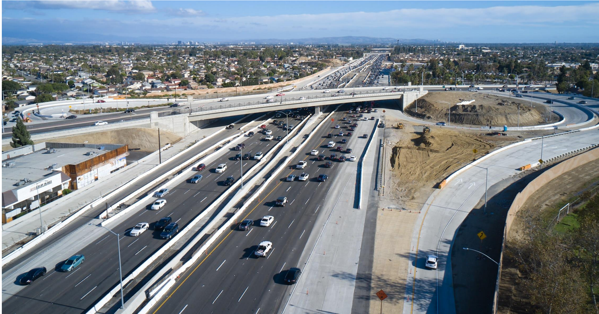
Mainline and ramp paving
