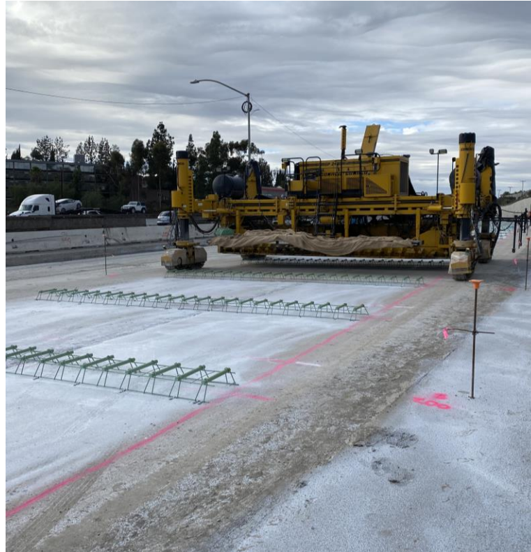
La Paz Road NB on-ramp JPCP Segment 2
