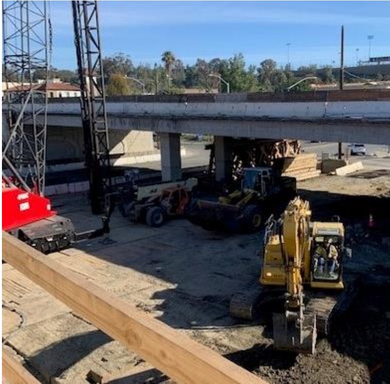
Avery Parkway stage 2A pile driving Segment 1
