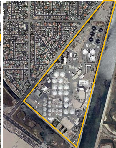
Treatment Plant No. 2 Huntington Beach
