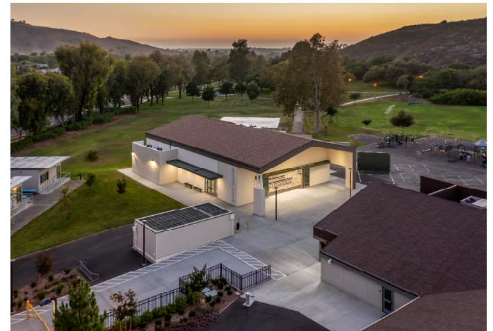
Bonita Canyon ES New MPR Building
