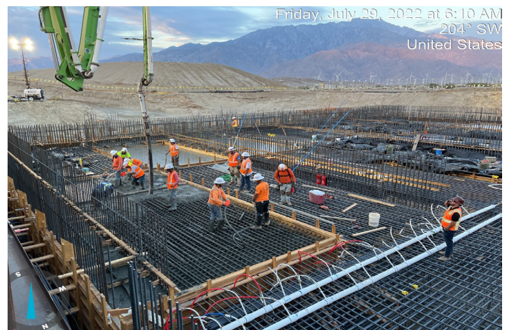
Above: Regional Water Reclamation Facility, July 2022
