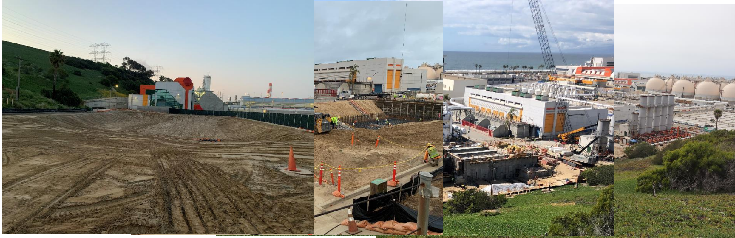
April 2020 – Site Preparation Complete September 2021 – Ductbanks and RNR Station Girders March 2022 – Areas under construction August 2022 – Current Progress
