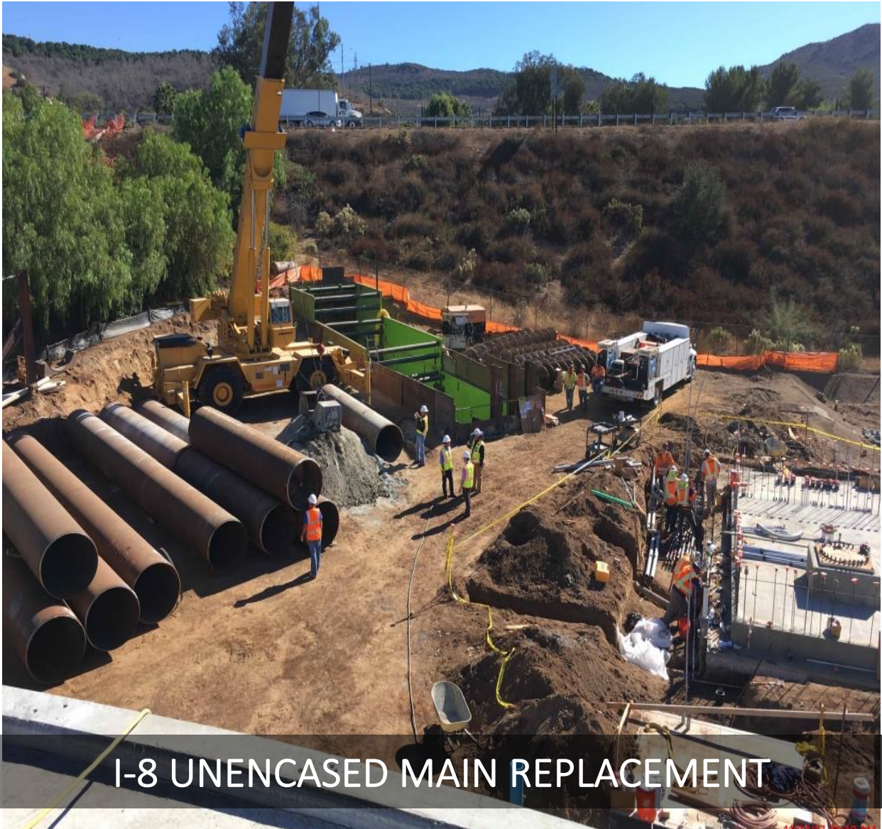
PIPELINE REPLACEMENT AT BRIDGE CROSSINGS
