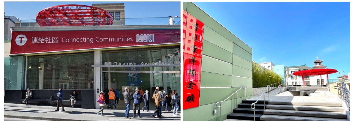
SF Central Subway Chinatown-Rose Pak Station
