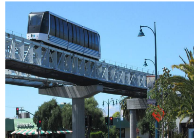
Cable Pulled Vehicles Manufactured by Doppelmayr
