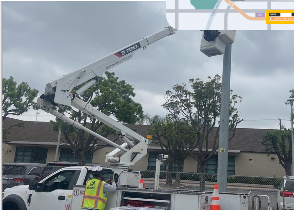
Installation of hardware
