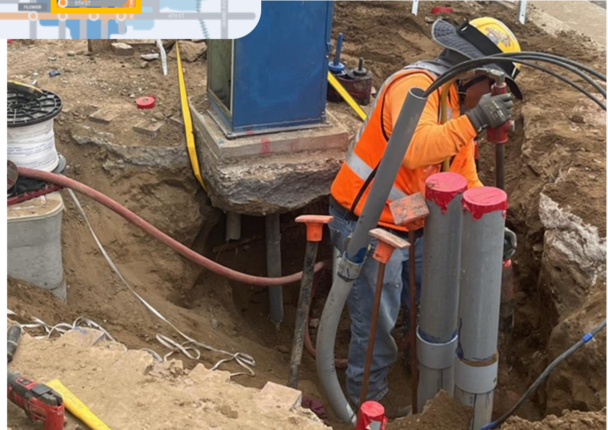
Forming traffic signal foundation
