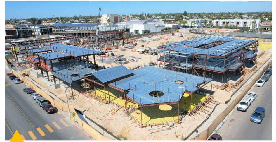
Central Elementary School - New Campus
