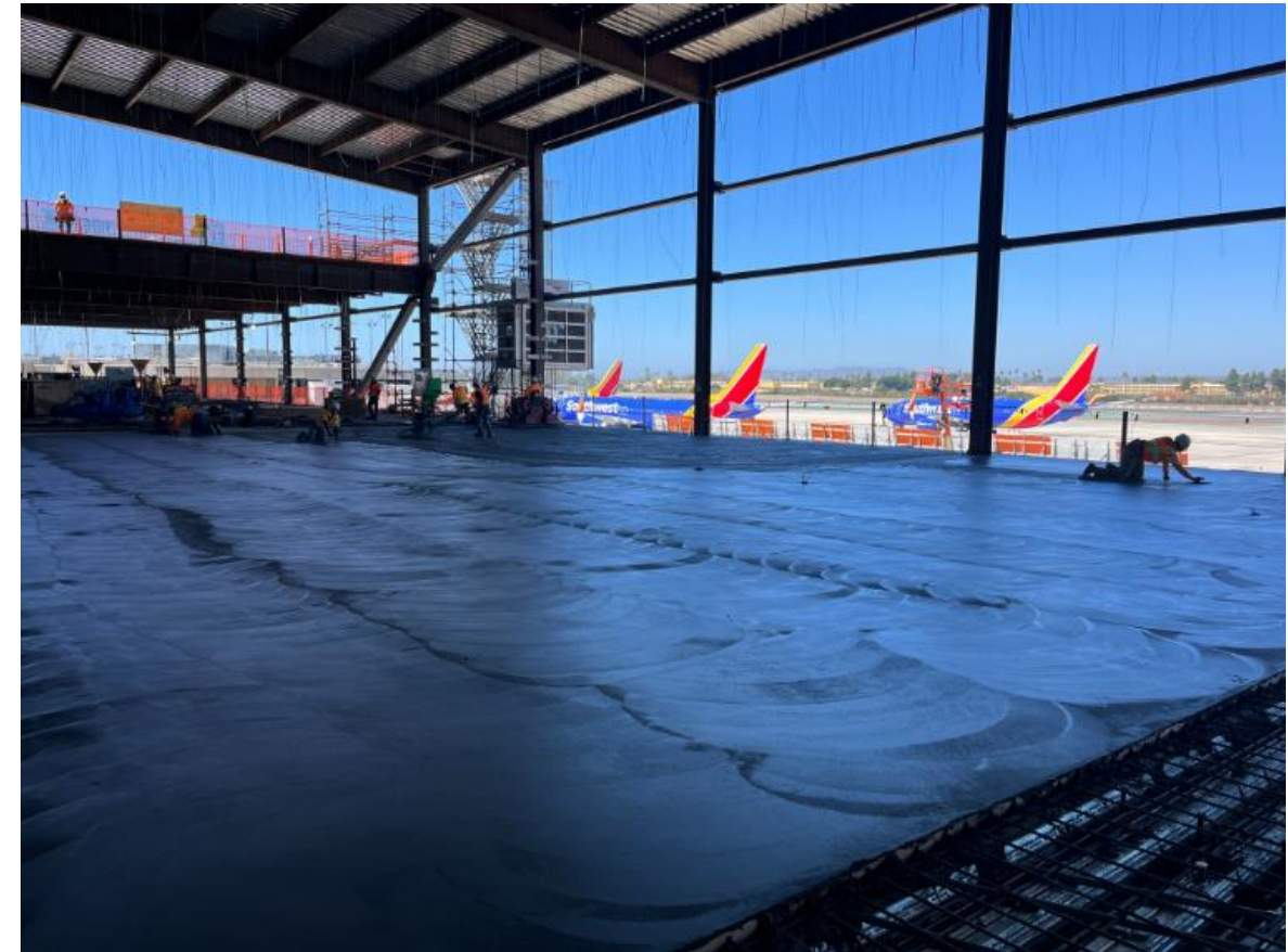
Concrete Finishing on Metal Deck in Progress
