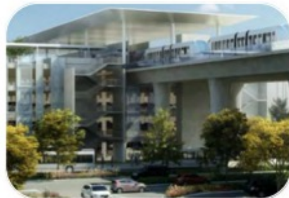
Consolidated Rent-a-Car Facility (ConRac)
