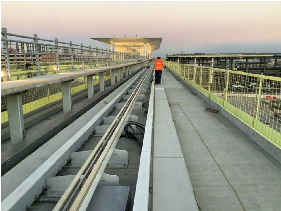
Guideway approaching ITFE Station
