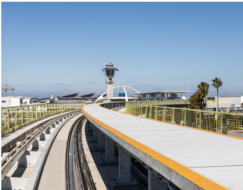
Guideway approaching CTA East Station
