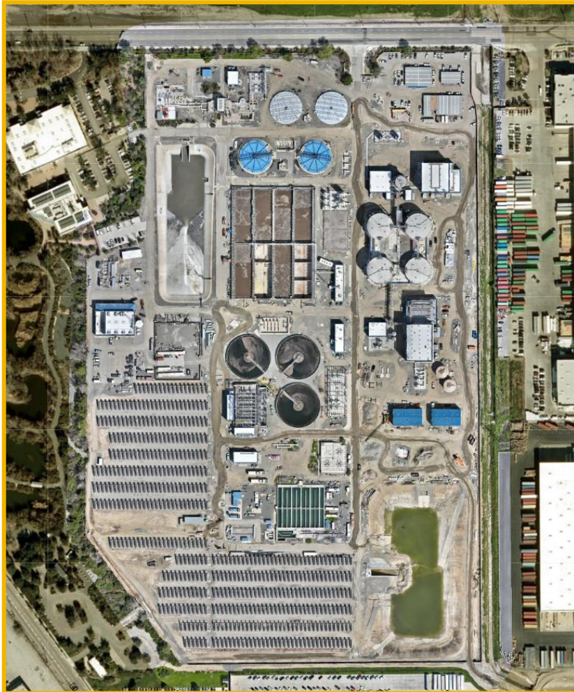
Regional Water Plant No. 5 City of Chino
