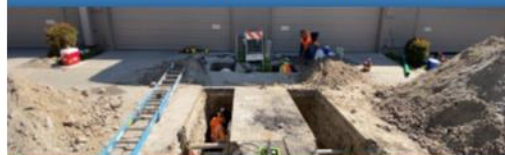
AC Water & Sewer Group Job 1051
