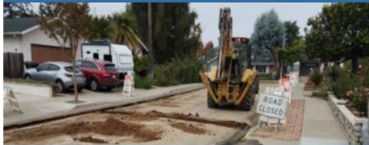
AC Water Group 1059
