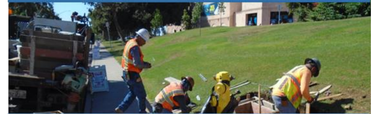
Balboa Park Pipeline Replacement Phase 2
