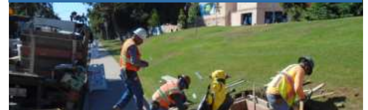
Balboa Park Pipeline Replacement Phase 2
