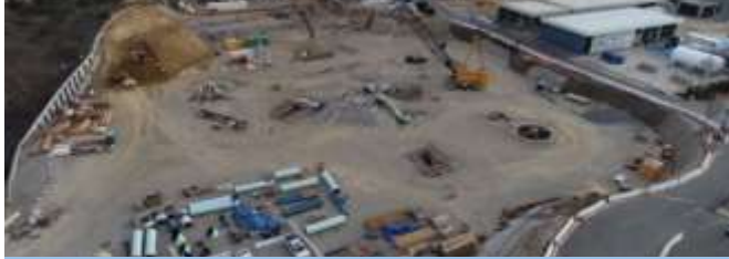
North City Water Reclamation Plant Grading
