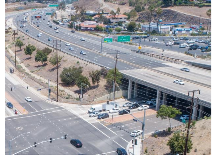
New Bridge over Lincoln Avenue
