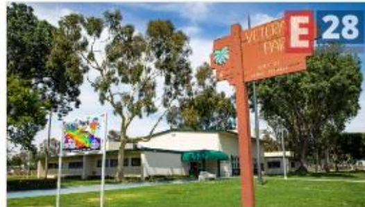
Veterans Park Roof Replacement
