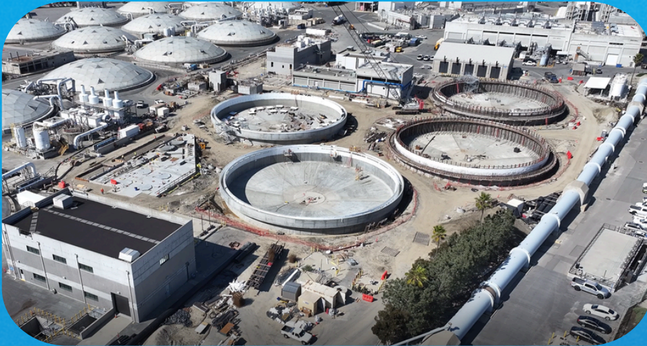
Project No. P2-98A is currently constructing four new Primary Clarifiers at Plant No. 2 located in Huntington Beach.
