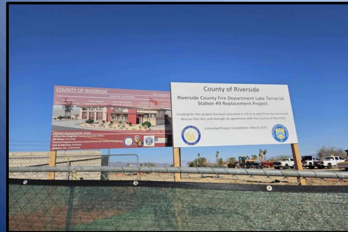
Grading and Demolition
