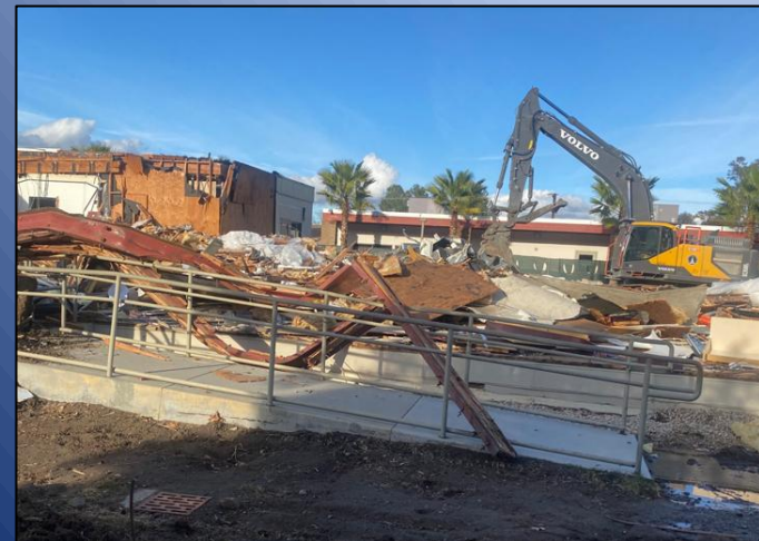
Existing Building Demolition
