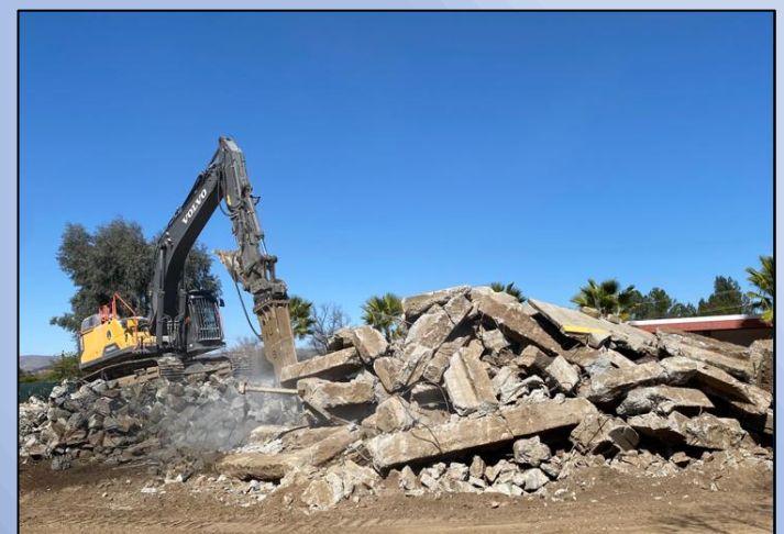
Concrete Foundation Demolition
