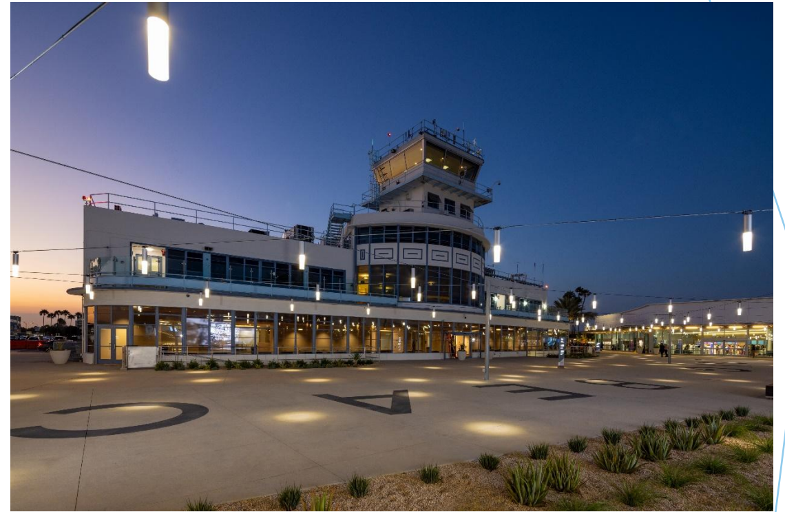
Restored exterior and opened west face
