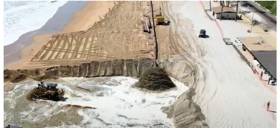
Pictures from City of San Clemente Sand Replenishment Project
