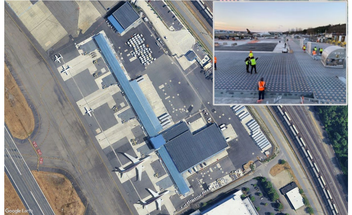
Through-the-Fence - UPS New Facility at Boeing Field
