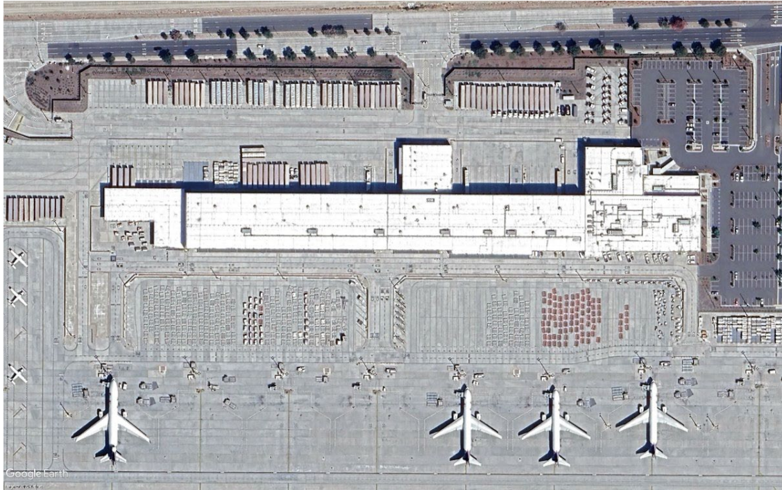
Sort Facility - FedEx New Facility at Ontario International Airport
