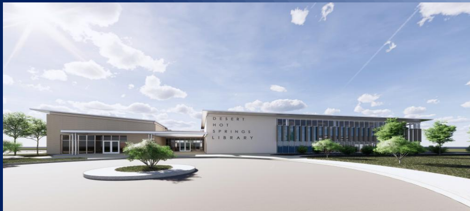
Riverside County Library System, Desert Hot Springs Library Project Value $13,000,000 Project Size: 15,000 SF LEED Silver
